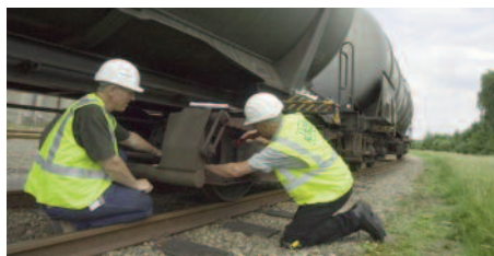
BRAKE BLOCK INSPECTION (SOURCE: LLOYD'S REGISTER RAIL)
