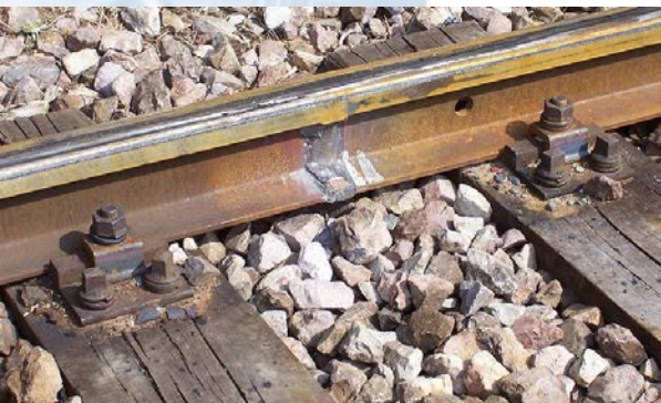
thermite weld
